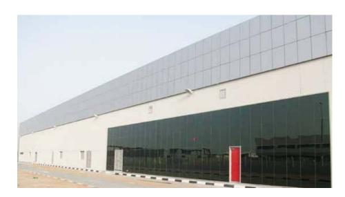
Al Rabiah Food Industries Warehouse, Office Building and workshop at DIP Second in Dubai. This was designed by EDMAC to tailor to the food industry requirements such as processing and packaging machines that require 15 meter high internal ceilings. This was funded by EIB and was delivered on time with full Client satisfaction.
